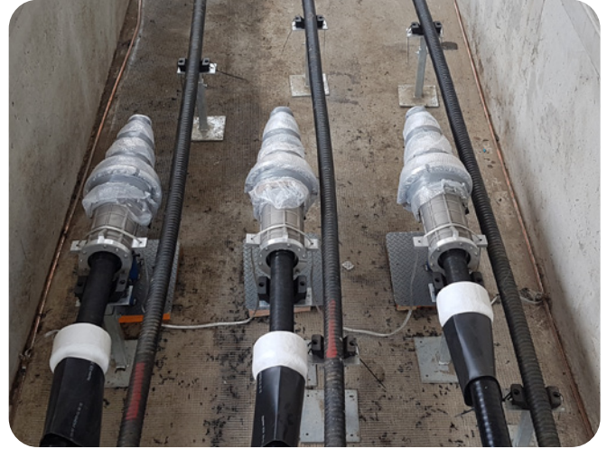
NKT 72.5-170kV Oil Transition Joint
