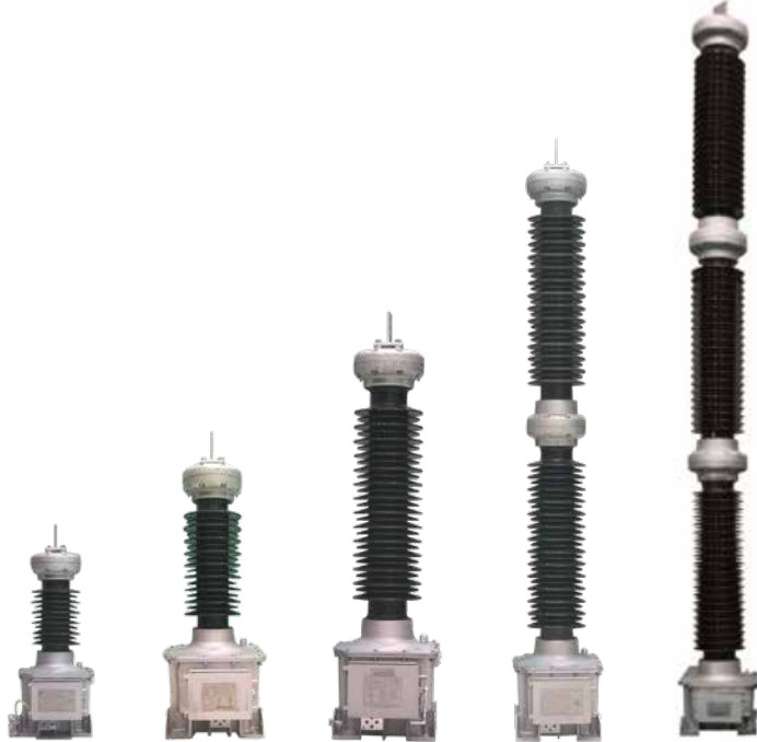
Capacitor voltage transformer
