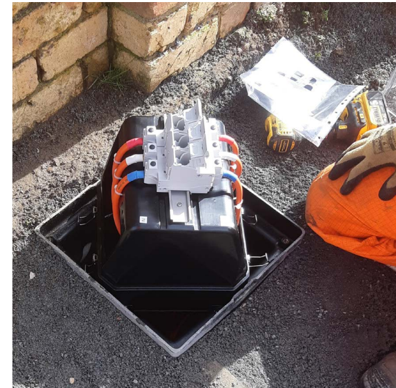
All service and maintenance work on a U-Pillar can be carried out safely above ground
