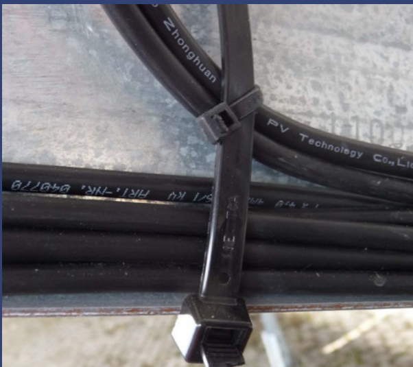
Fixing solar cables onto PV racking structure
