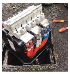
Pre-installed cabling allows the U-Pillar fusegear stand and the protective bell covering it to be lifted out of the pit for easy inspection and maintenance above ground – on both branching and looping networks
