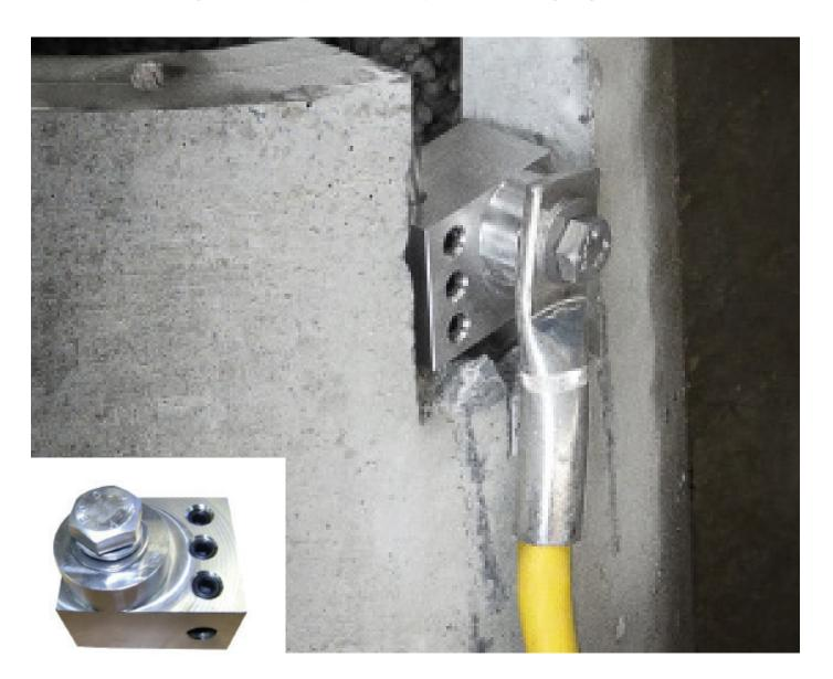
The Hiko REBAr provides a secure means of bonding the internal reinforcing cage of older hollow spun concrete poles to the external copper cable earthing system.
